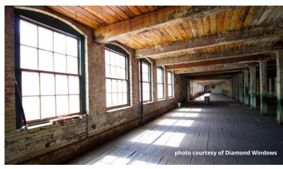
**Pictured above:** Existing masonry was repaired, and the former factory's massive interior timber beams and large window openings were preserved.
